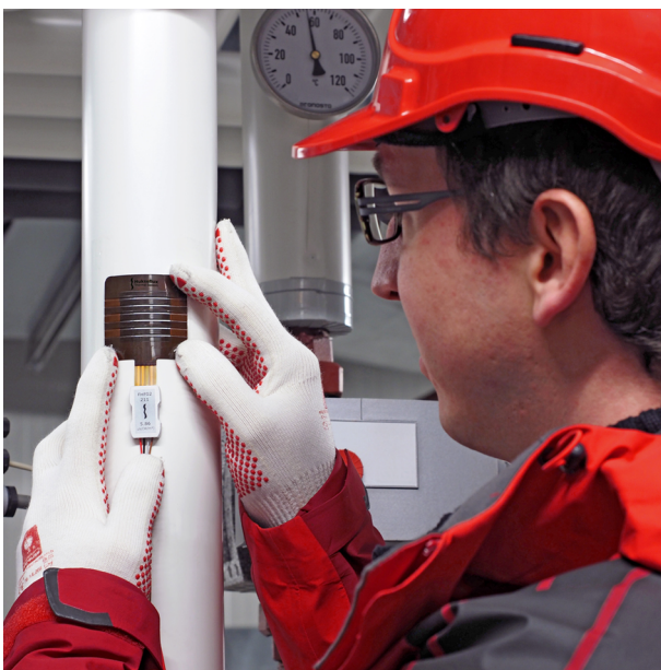
Figure 2 FHF02 being installed on a pipe
